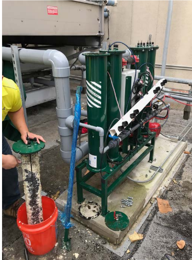
Figure 1. Scraping scale off the reactor rod of the electrochemical water treatment system.
